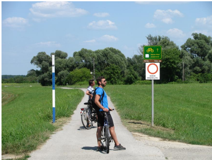
Figure 14: Asphalt paved flood protection dike, as bicycle path between Felsőszentmárton and Drávasztára.
