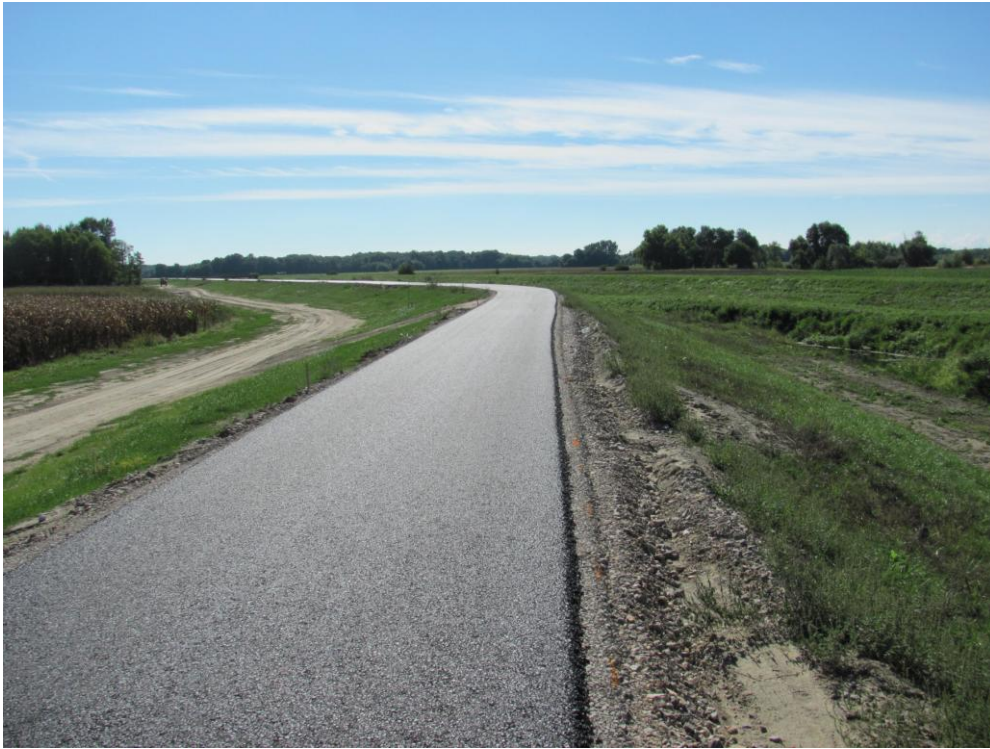
Figure 6: The Ancient Drava bike route under construction.
